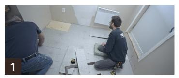
Before beginning the installation, **measure the dimensions of your flooring project in inches** because the *Ekösteps*® insulating tiles are squared to inches. Divide length and width of the room by 24 in (width of each Ekösteps® insulating tile) in order to determine the number of tiles required per axis. It is frequent that each row's last tile and the ones of the last row will need to be cut.
